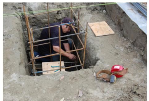
Carpenter tying the steel footing dowels for the steel columns canopy
