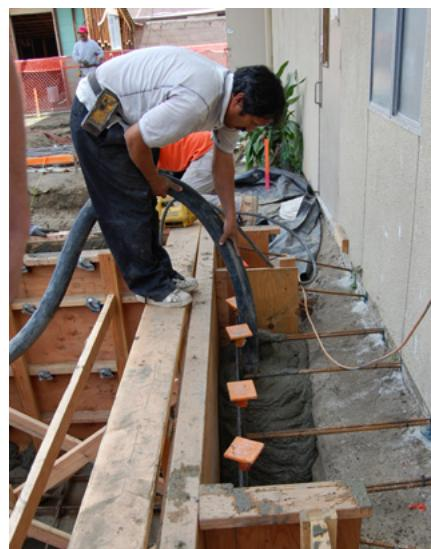
Pouring the elevator pit walls and footings
